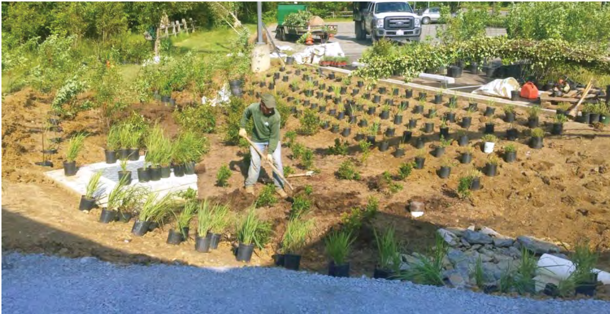
Figure 23: Stormwater infrastructure construction (Source: http://thecleanwaterpartnership.com )
