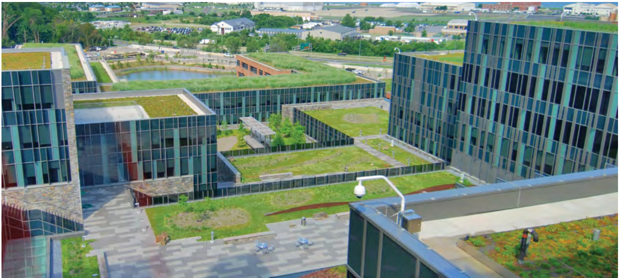
Figure 22: Green roofs, US Coast Guard HQ (Source: http://www.gsa.gov/portal/content/166443 )
